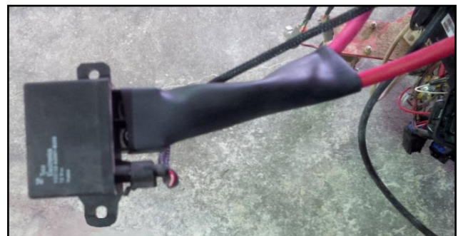
Figure 13 - Heat Shrink over exposed wires/posts
